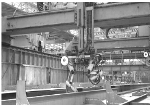
Fig. 1 Robot welding shop for subassembly
