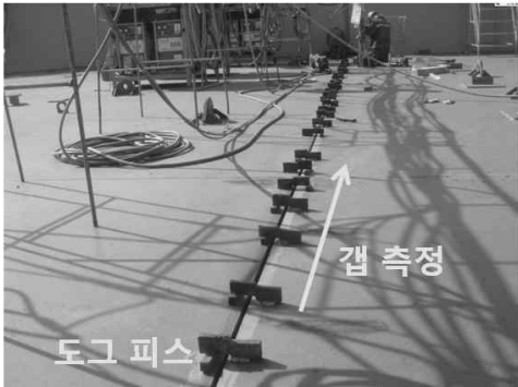
Fig. 2 Alignment of 1G welding joint
